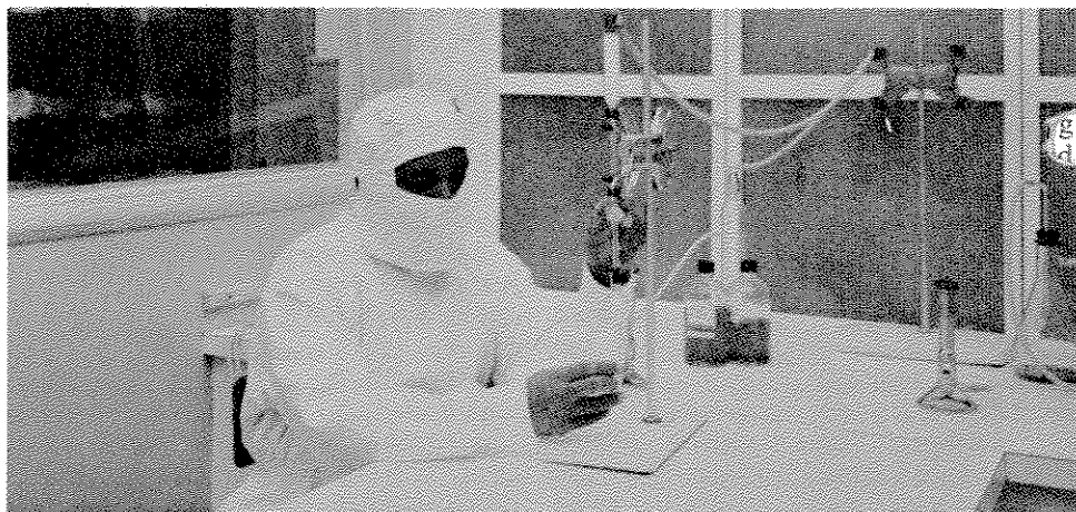
Lartius Dupree carries out an experiment in the newly developed clean rooms at Shirley Research. The air enters through the absolute filters (at right in picture), circulates around the worker and his instruments, and then up and out of the room.
