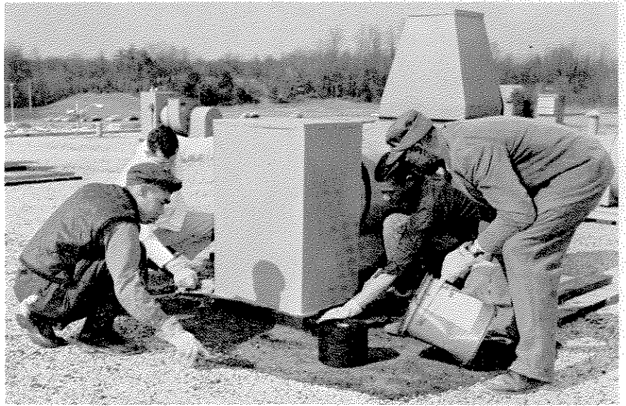
THOUGH APRIL SHOWERS MAY COME OUR WAY, the roof should withstand them. Here (left to right) Roscoe Newman, William Pickering, Wilbert Ewell, and Chauncey Johnson repair the flashing around a vent on the roof of the Falls Church plant.
