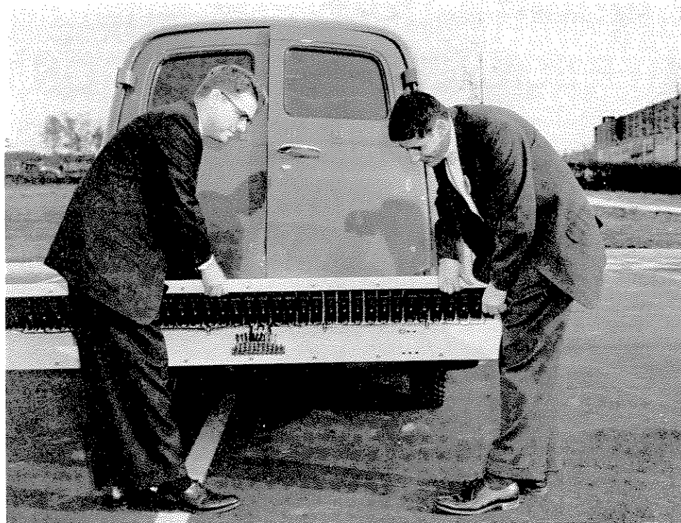
REAL CRAZY BUMPER —Melpar's Special Products Department Manager, Emmett Bradley and Bureau of Public Roads Research Psychologist Dr. Richard Michaels adjust the Road Eye—a Lateral Displacement Detector which will measure normal driving deviations in a new BPR highway research program. Study will include tests to determine subconscious affect near the highway on "swerve and curve" control. Roadeye was developed by Melpar's Special Products Department to the Bureau's specifications.
